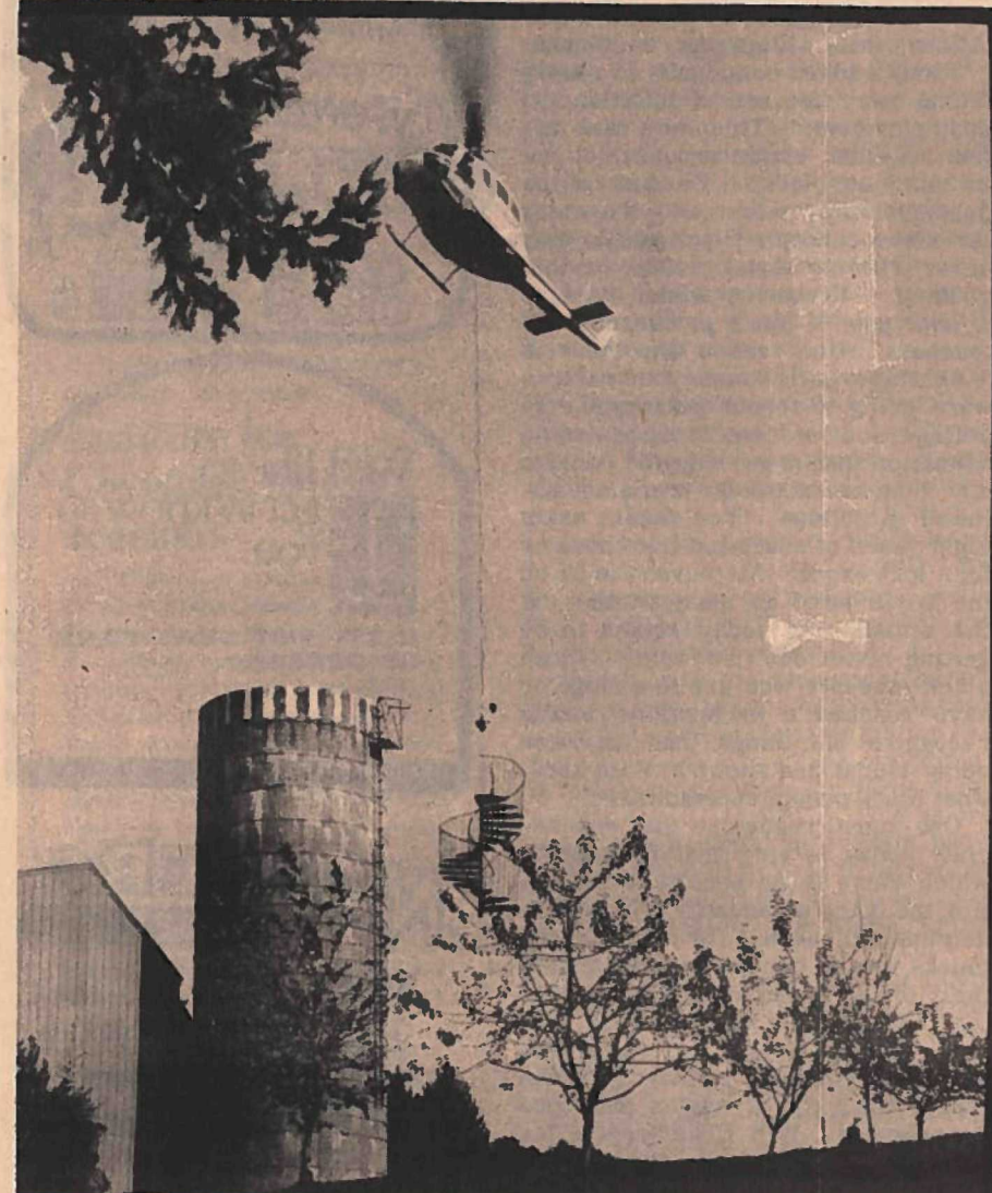
Donating the time, an Evergreen helicopter here lowers a piece of a spiral staircase in the Tilikum Silo. It will soon become an observation tower (How do you like them oats?)
